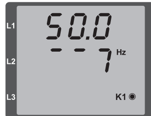
Example 1: Fig. Display of the mains frequency (50.0 Hz) and the phase sequence.
