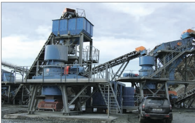
Image 2: Practical example for flicker: Gravel quarry
