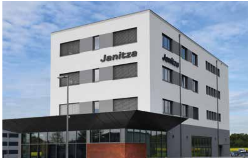
Headquarters: Lahnau, Germany.
